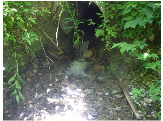
Photo 50 Station 10-27 – Unnamed water body – Facing upstream (south) on north side of McKay Road – perched culvert.
