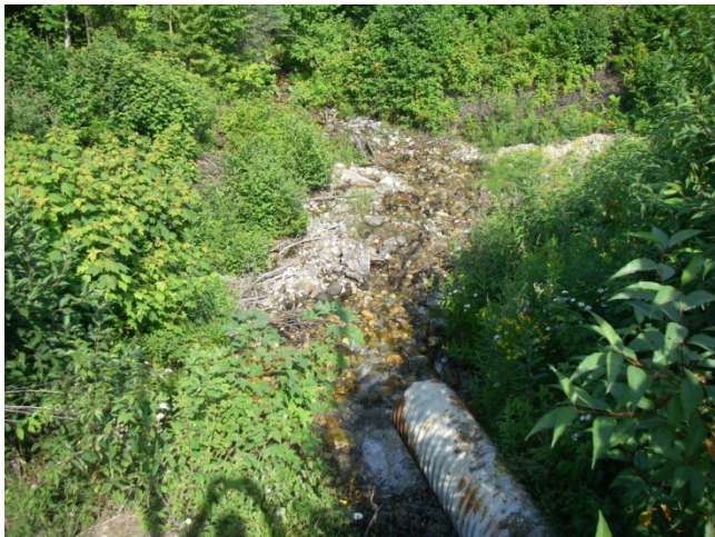
Photo 33 Station 9B10 – Unnamed water body – Facing downstream (west) showing water body channel and a perched culvert.
