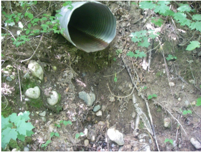
Photo 7 Station 0-1 – Unnamed water body – Showing perched downstream culvert.
